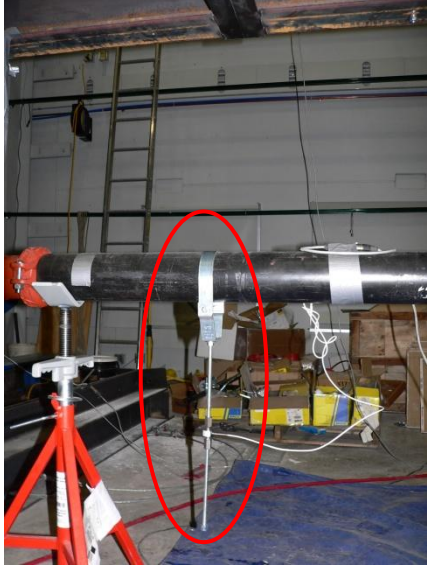
(a) Vertical hanger sheared off (Configuration 3-5, 100% MCE level)
