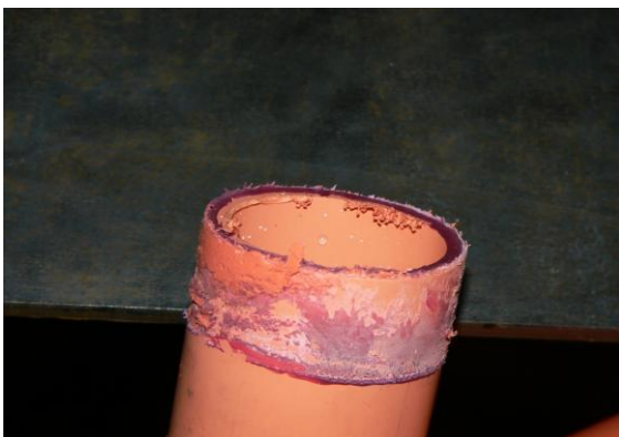
Pipe pulled out from tee joint
