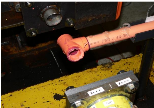
Pipe pulled out from tee joint
