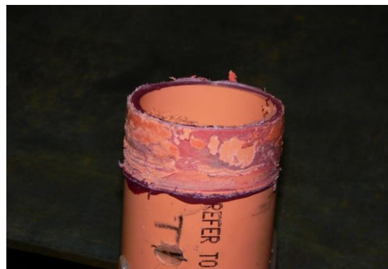
Pipe pulled out from tee joint
