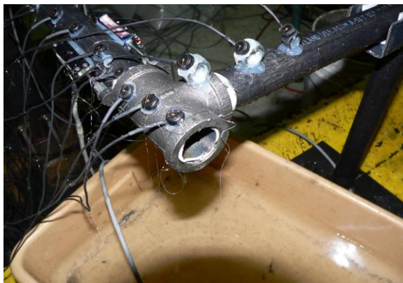
Pipe fractured at the edge of tee
