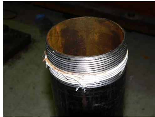
Pipe threads damage
