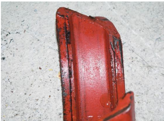
Coupling flange fractured
