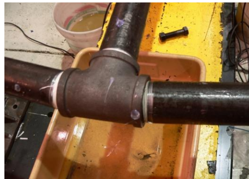
Pipe threads slip from tee threads
