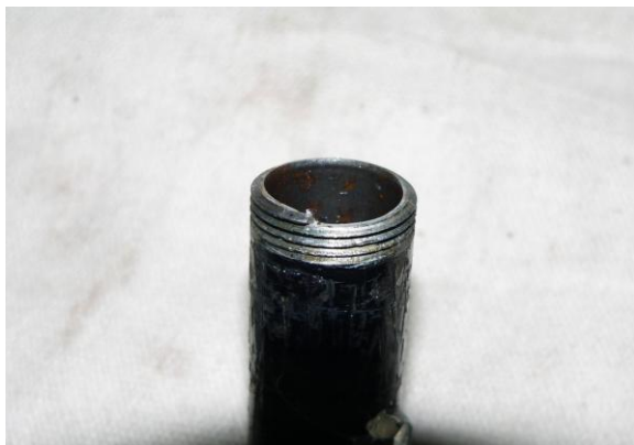
Pipe threads erode due to imposed rotation
