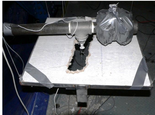
(a) Damage of flexible ceiling box (Configuration 1-6, 100% MCE level)
