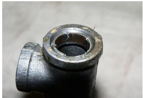
Pipe fractured at the edge of tee
