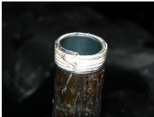
Thread sealant (Teflon tape) degraded
