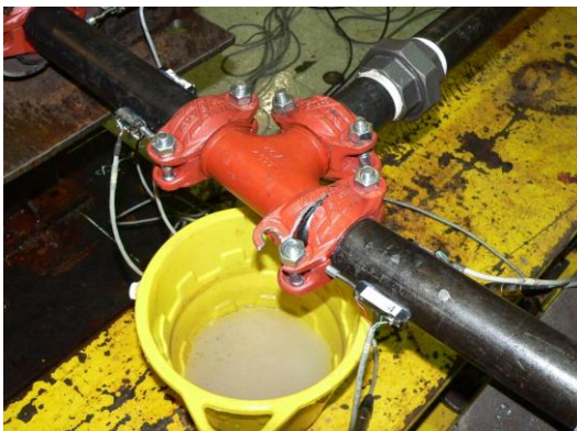
Flange coupling fractured
