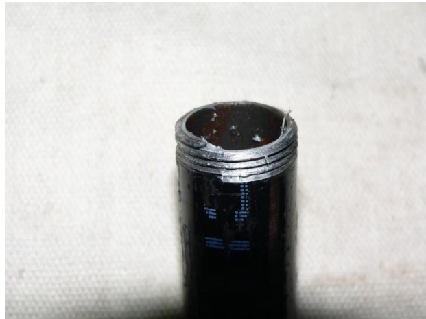
(f) Sheared threads in the pipe
